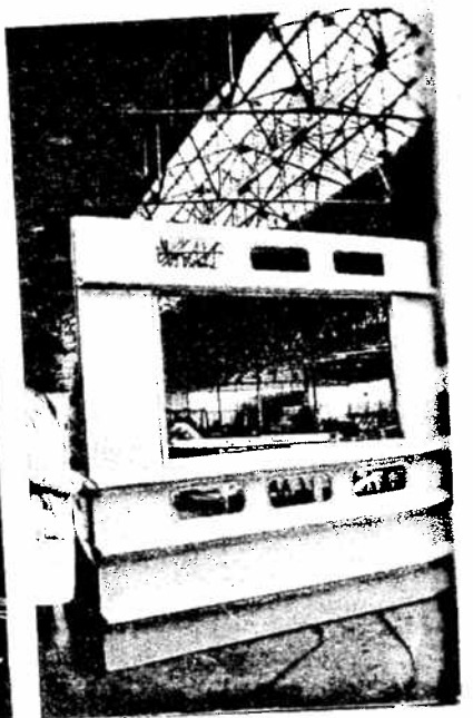
Fig. 25. Examples of prefabricated aluminum panels devised by Jean Prouvé Source: L'Architecture d'Aujourd'hui, February 1955
