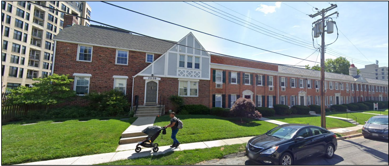
Figure 2 – View of Subject Property from Strathmore Street
