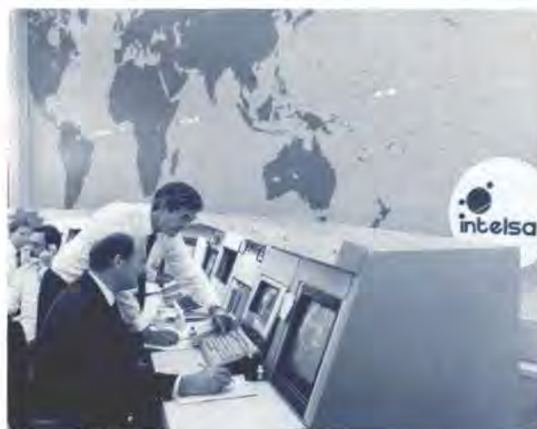
Figure 3. The INTELSAT Operations Center TDMA Facility provides centralized monitoring and control of TDMA satellite communications networks
