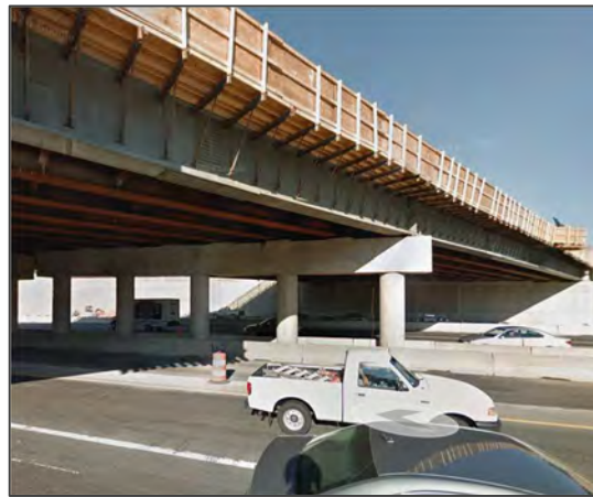
Figure 2: With New Bridge Structure (2011)
