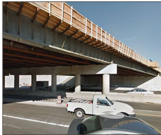
Figure 2: With New Bridge Structure (2011)
