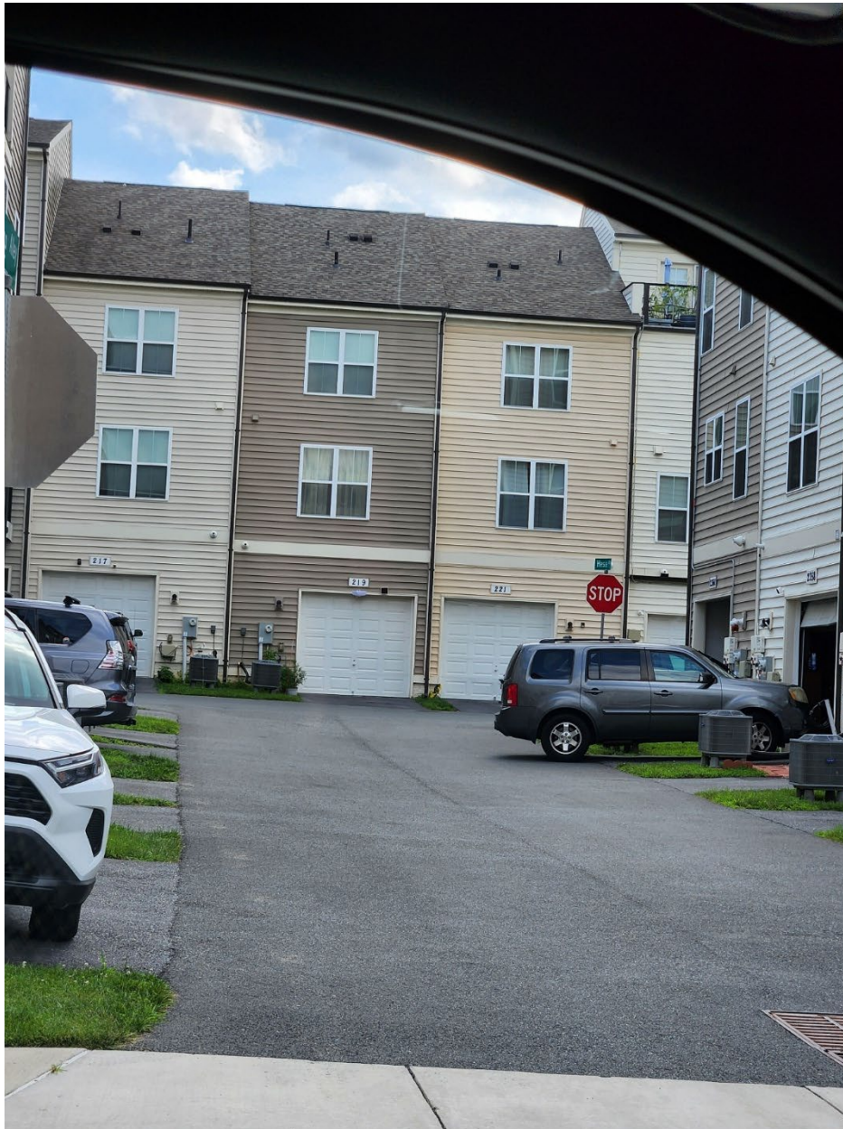
Figure 5. Lack of Unit Parking Space
