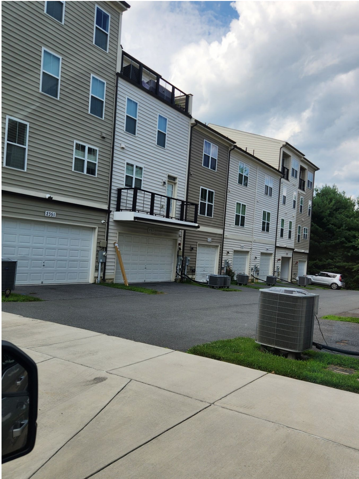
Figure 4. Parking in Back – lack of space
