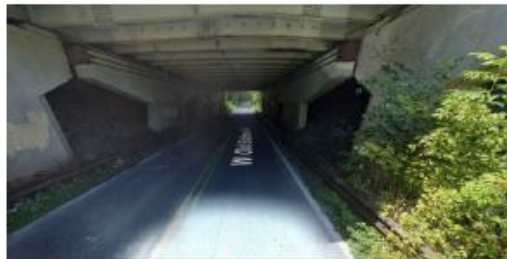
CURRENT CONDITION - WEST OLD BALTIMORE RD UNDER I-270
