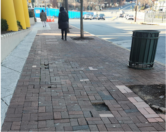
The existing brick sidewalks in Silver Spring need constant maintenance, with missing bricks causing unsafe conditions for pedestrians (left). On Georgia Avenue, a recent streetscape project allowed the Urban District to install a poured-in-place concrete sidewalk to indicate a clear path for pedestrians (right).
