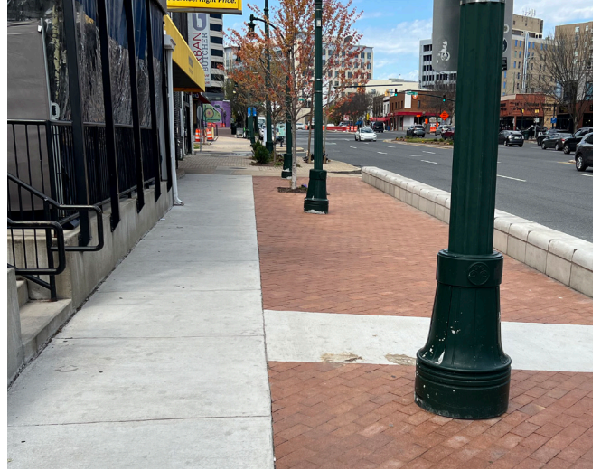
The existing brick sidewalks in Silver Spring need constant maintenance, with missing bricks causing unsafe conditions for pedestrians (left). On Georgia Avenue, a recent streetscape project allowed the Urban District to install a poured-in-place concrete sidewalk to indicate a clear path for pedestrians (right).
