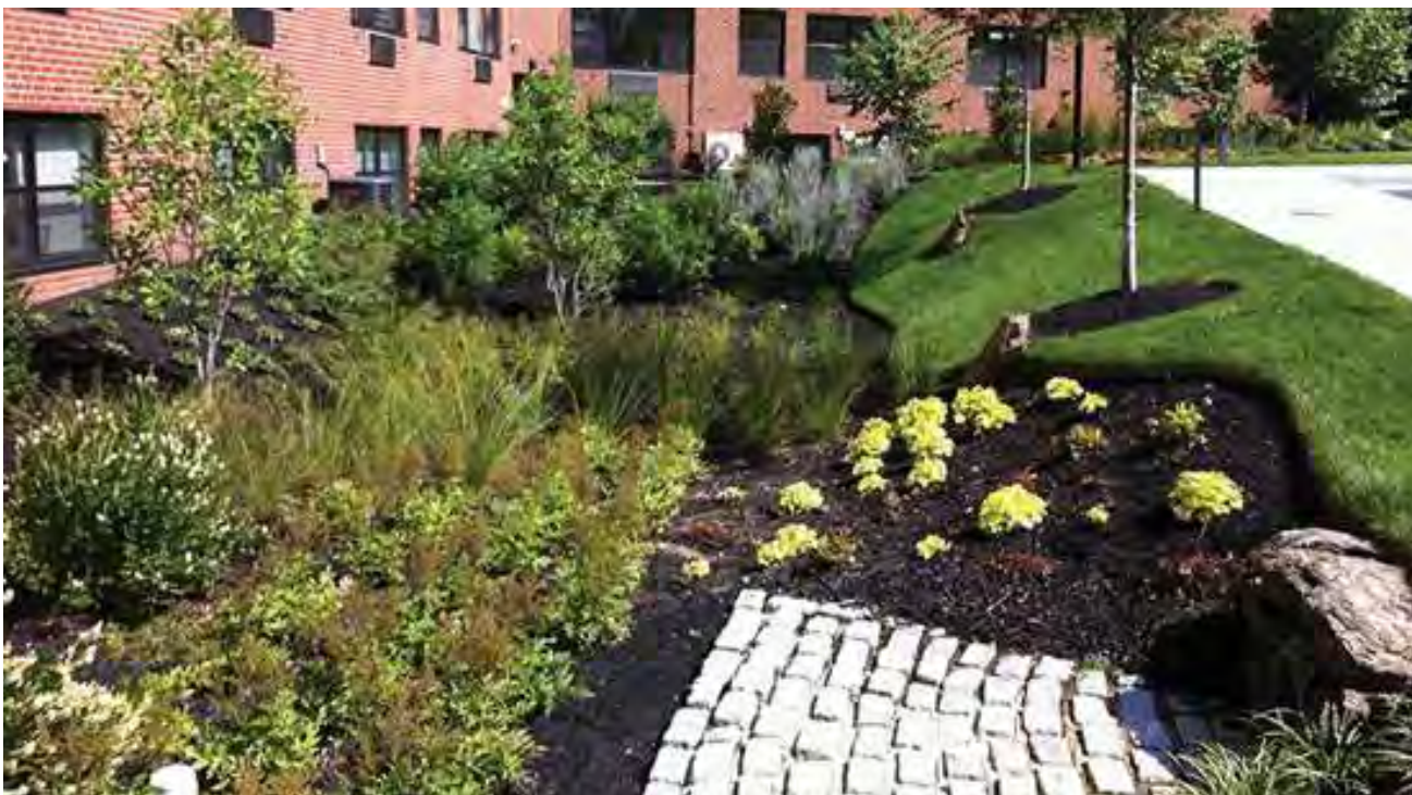
Figure 19: Micro-Bioretention Planting
