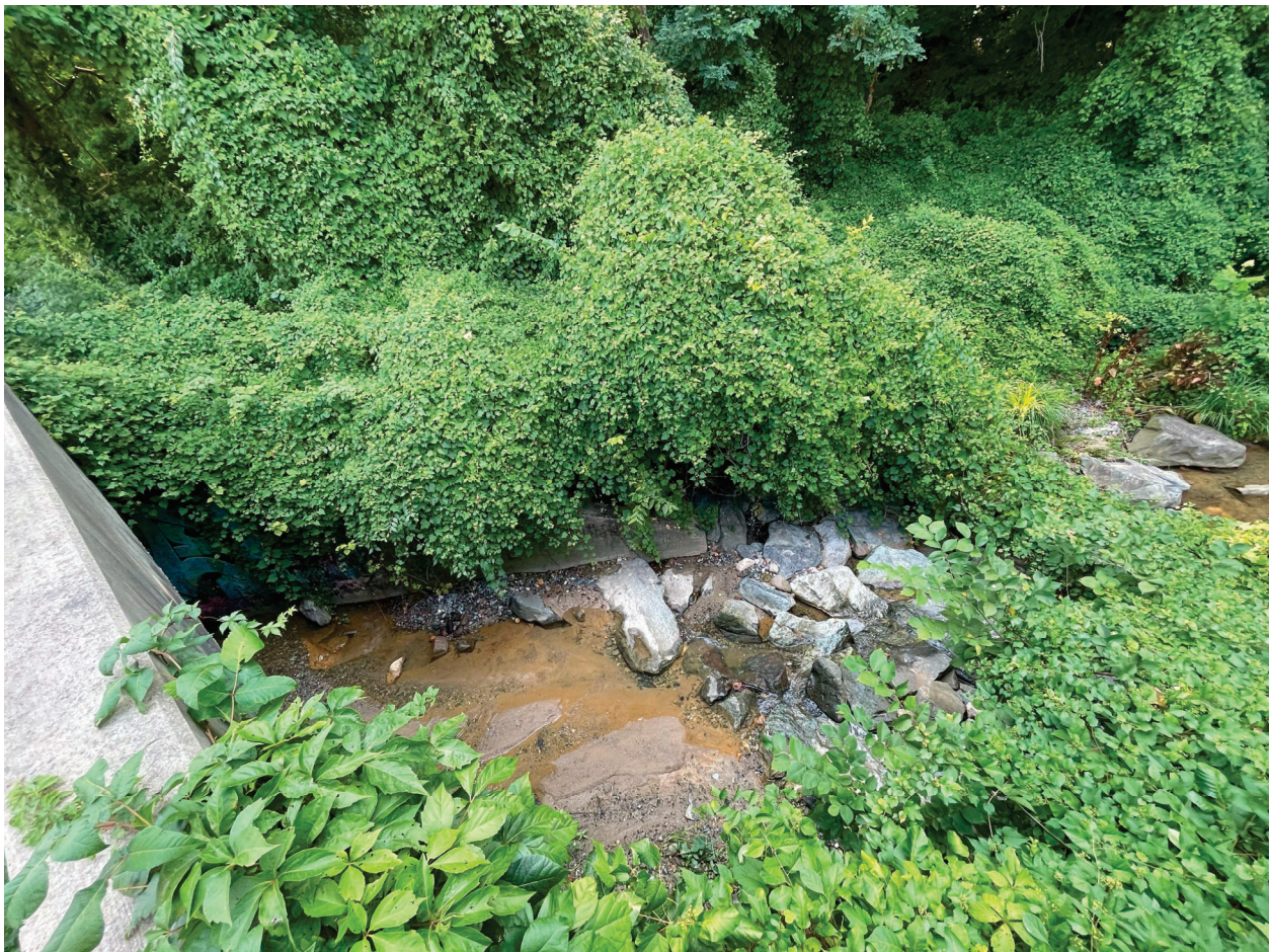
Figure 5: Looking at Outfall B
