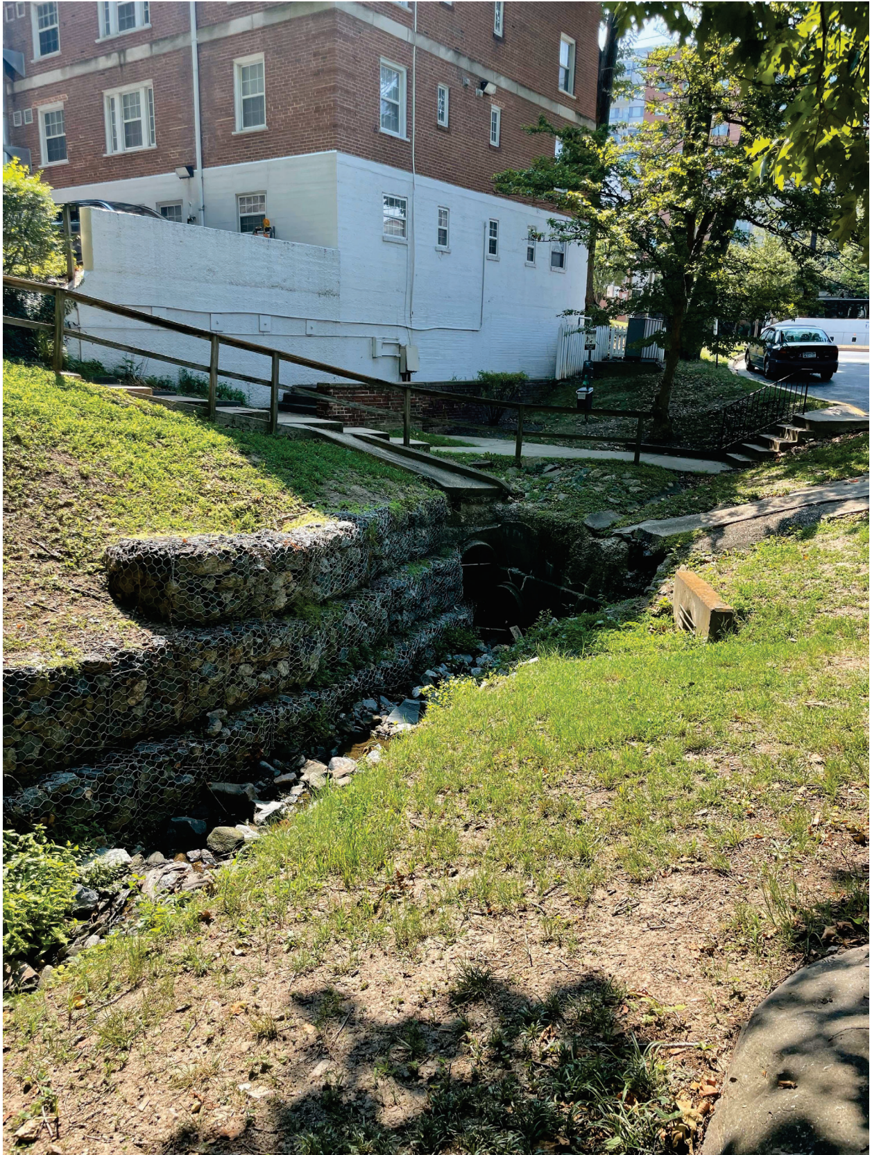
Figure 11: View of receiving pipe at downstream end of channel
