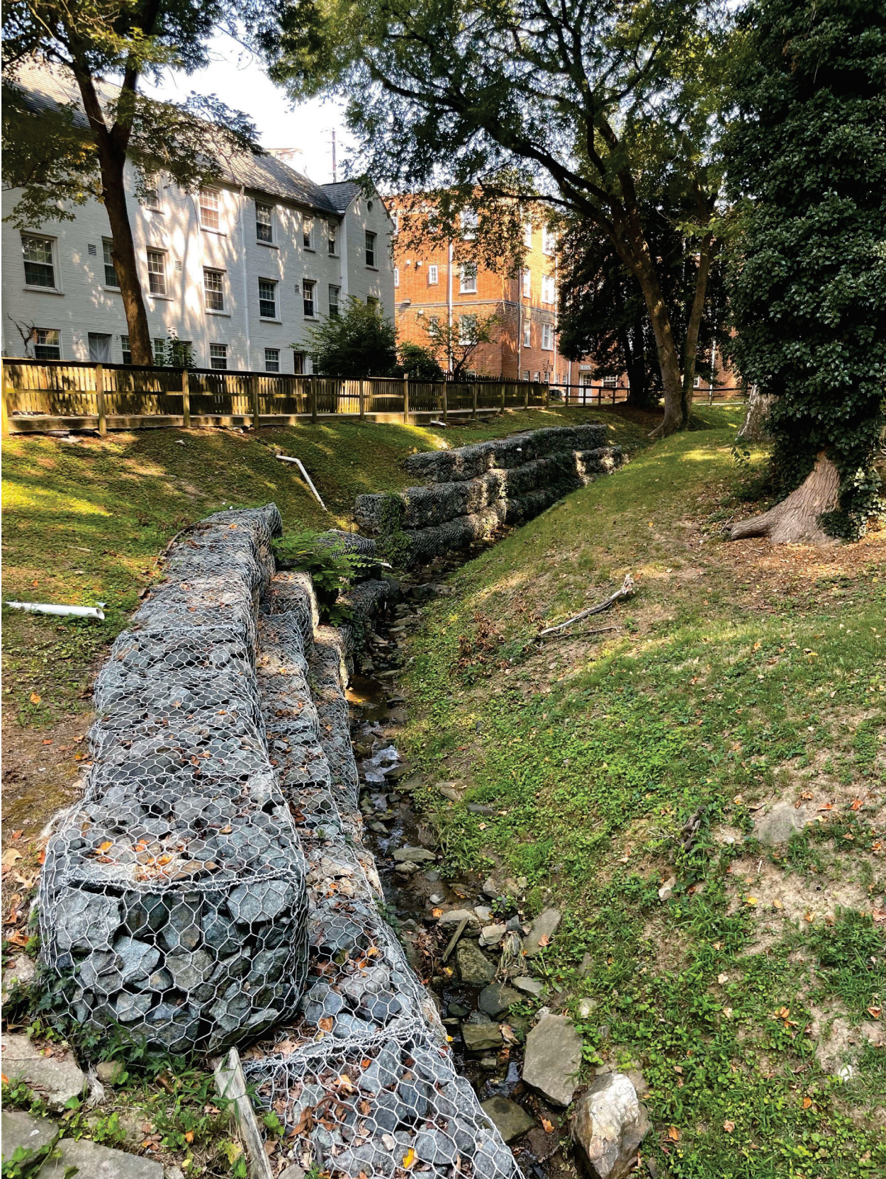
Figure 10: Looking upstream (north)
