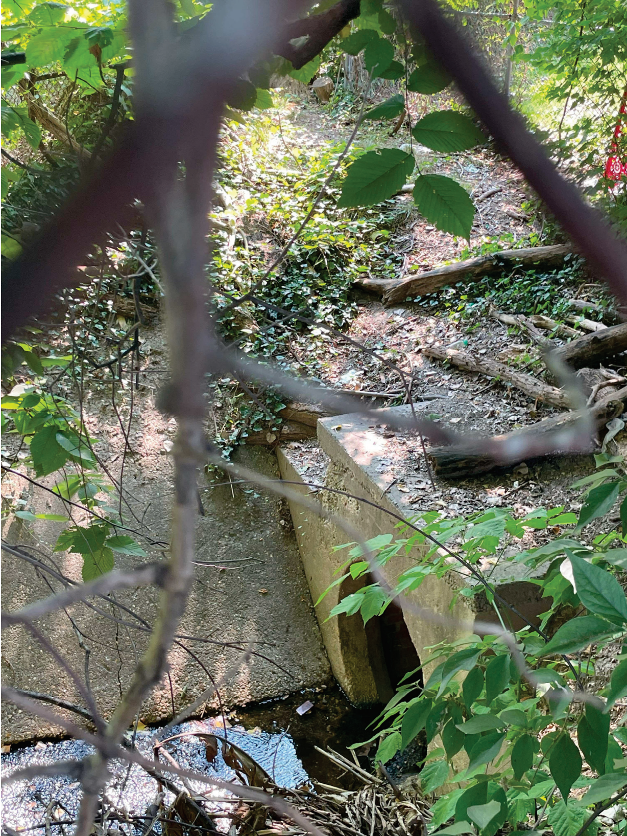
Figure 4: Looking at receiving pipe downstream of Outfall A
