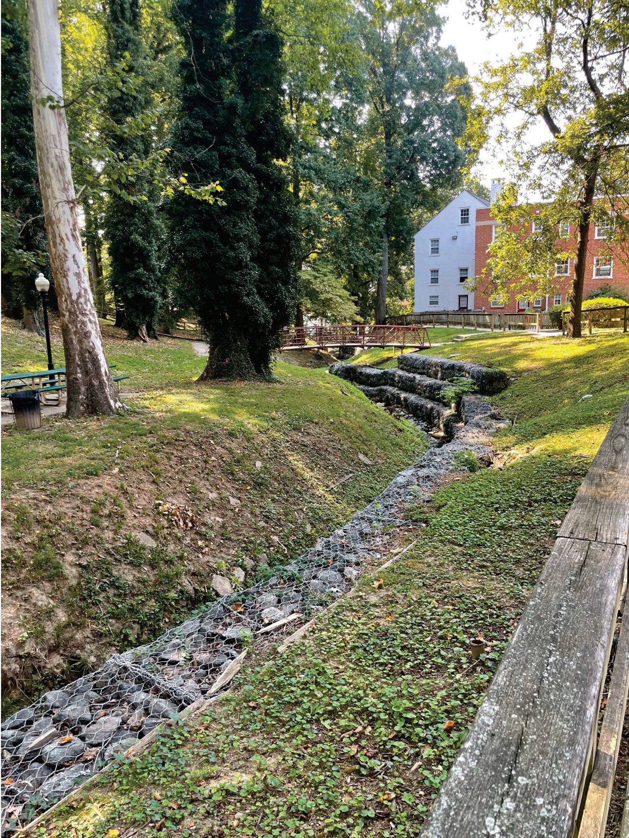
Figure 9: Looking downstream (south) of Outfall C
