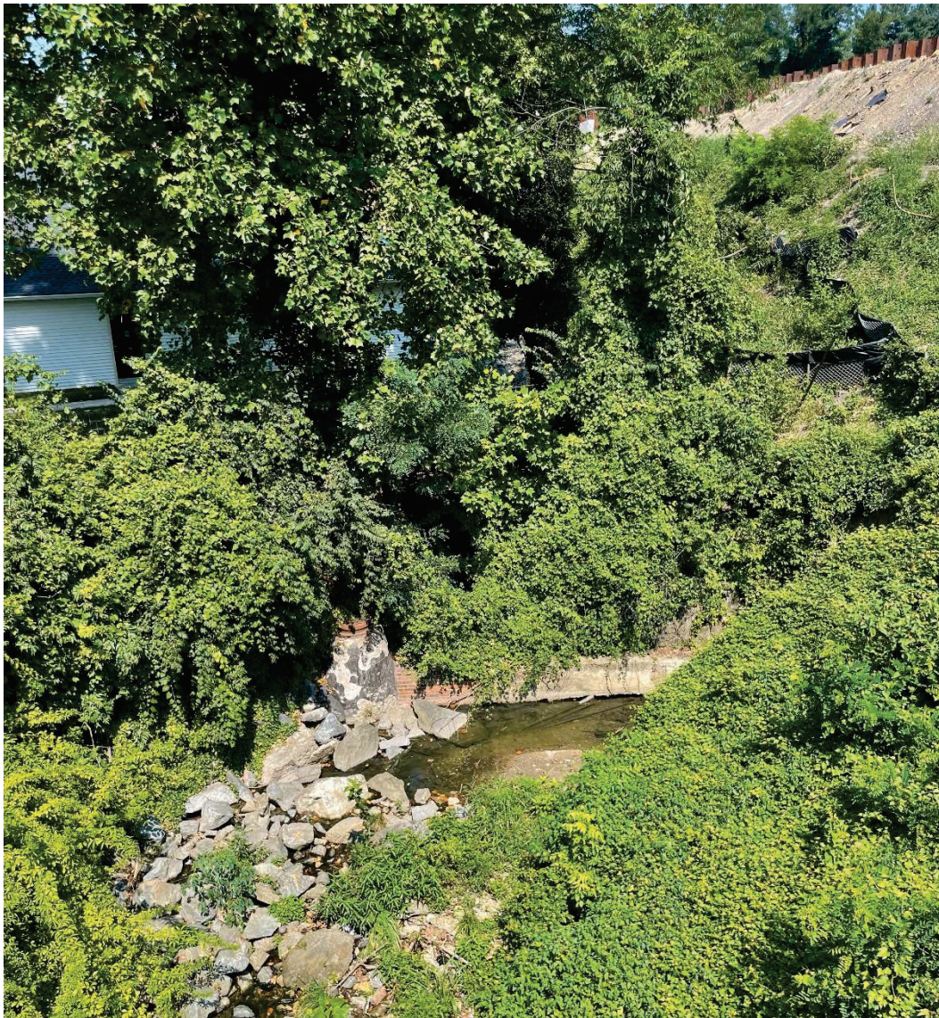
Figure 2: Channel immediately downstream of Outfall A.
