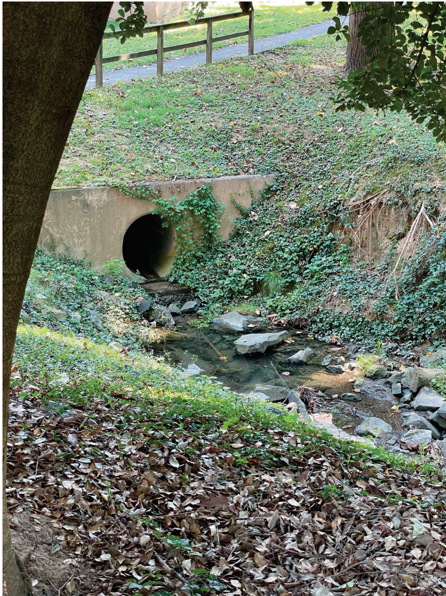
Figure 8: Looking at Outfall C headwall
