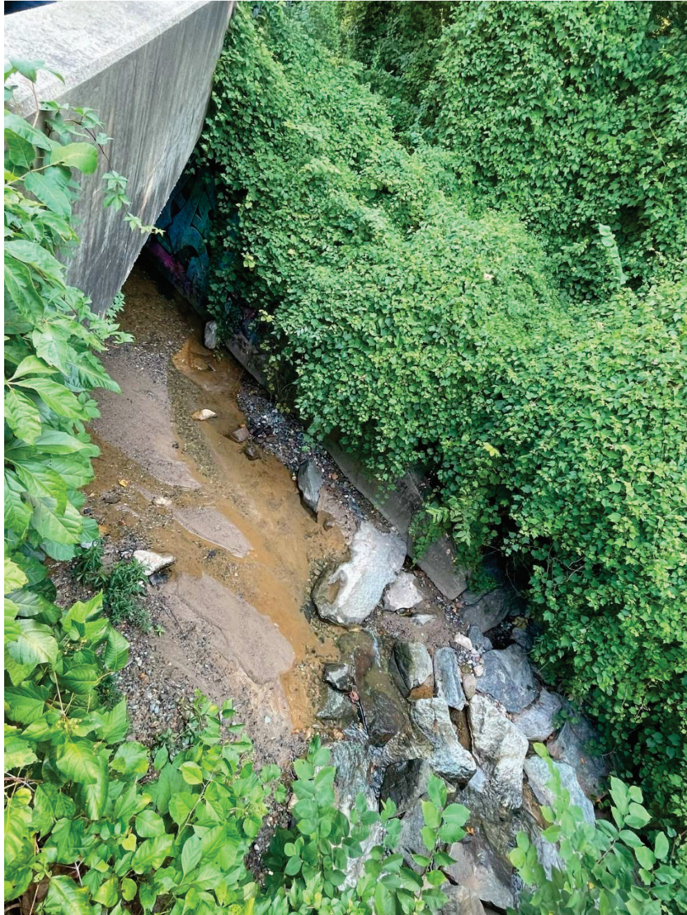
Figure 2: Receiving channel immediately downstream of Outfall B
