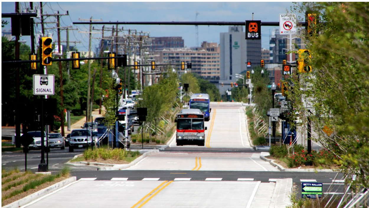
The Metroway BRT Service Operates in a Two-Lane Median Transitway
