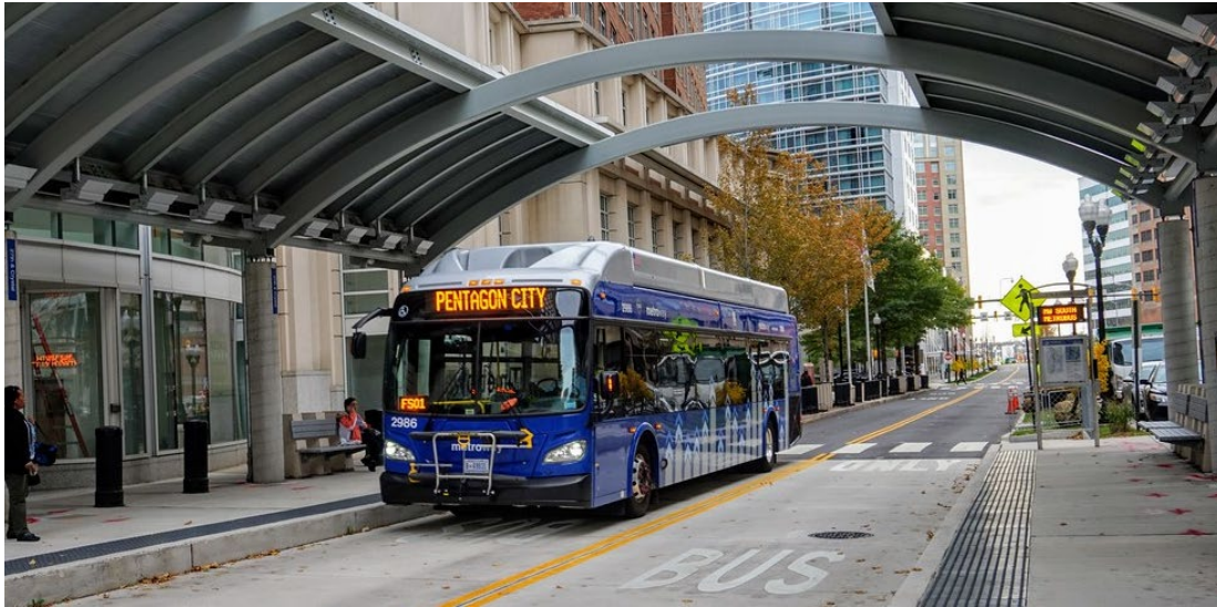
An Enhanced Station on the Metroway in Crystal City, Virginia
