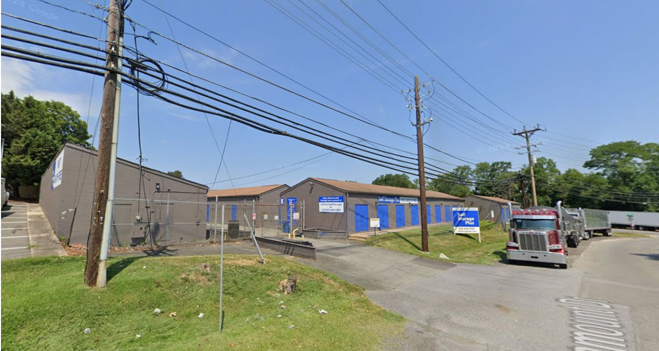
Figure 4: Street view from Paramount Drive, looking northwest.
