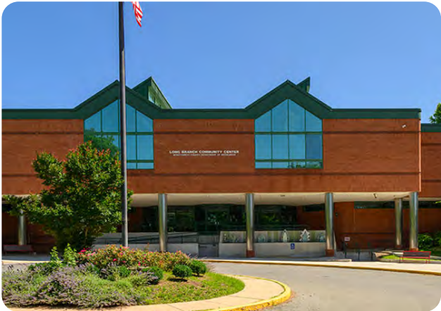
Long Branch Community Recreation Center
