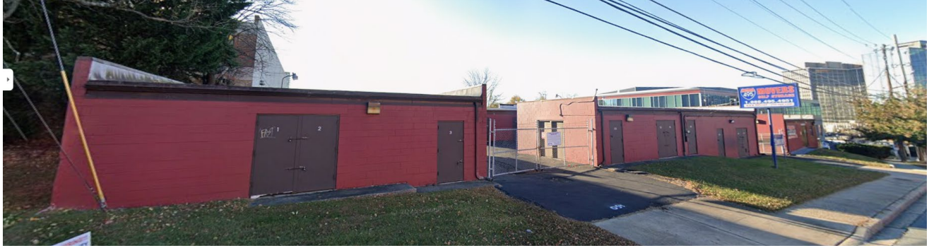
Figure 4: Streetview of Existing Conditions - Parklawn Drive
