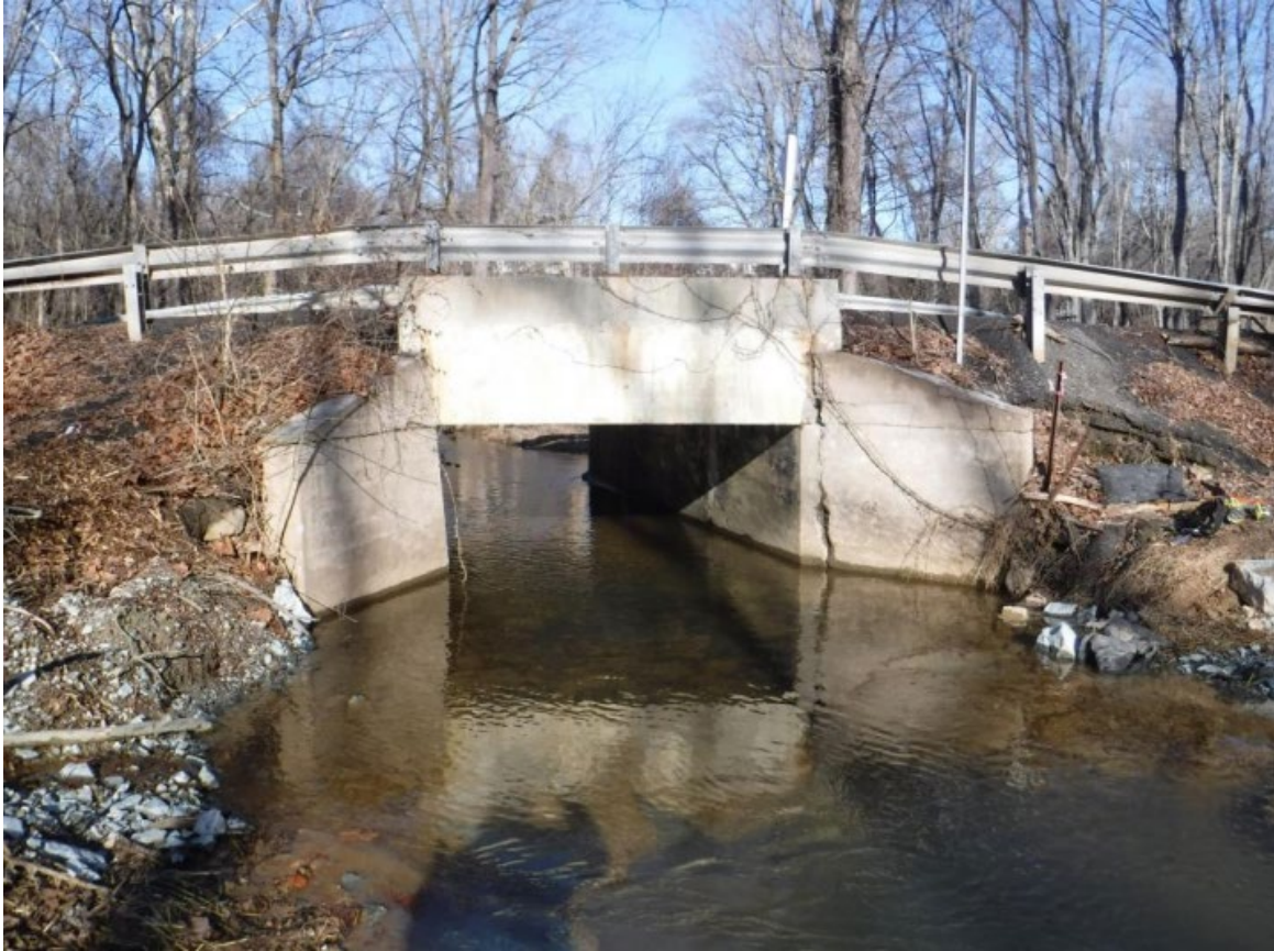
Figure 3: Existing Bridge Side View
