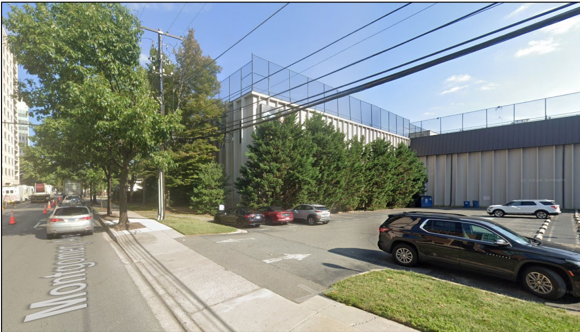
Figure 3 – View of the existing health club on Montgomery Ave. on the Subject Property
