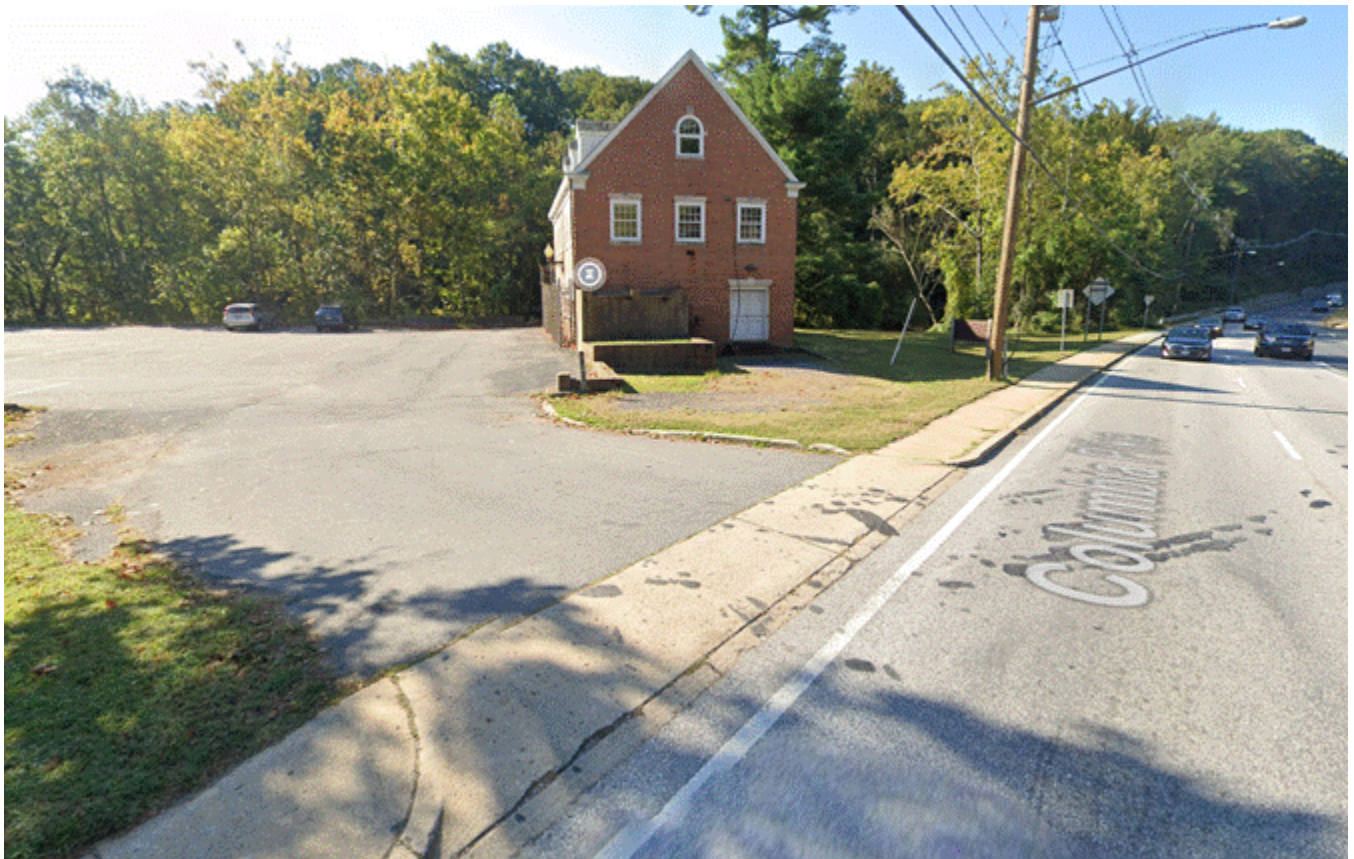
Figure 31: Street View Showing Existing Driveway Apron and Sidewalk
