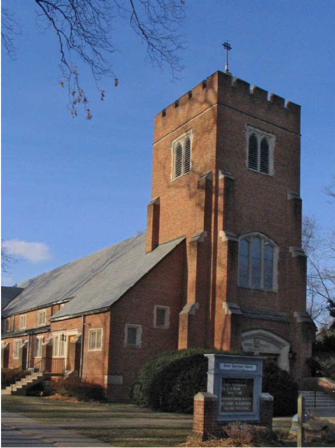
Figure 13: View of Grace Episcopal Church, 2020. Source: Montgomery Planning.
