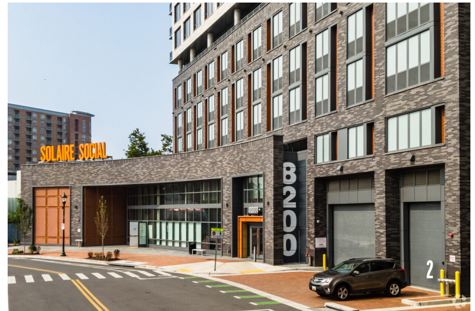
(1) M-NCCPC HQ, Wheaton, MD (2) Solaire Apartments, Silver Spring, MD
